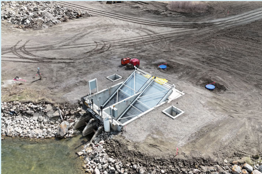
Lateral 61C Phase 2: Newly Installed Pre-Cast Screener Structure
