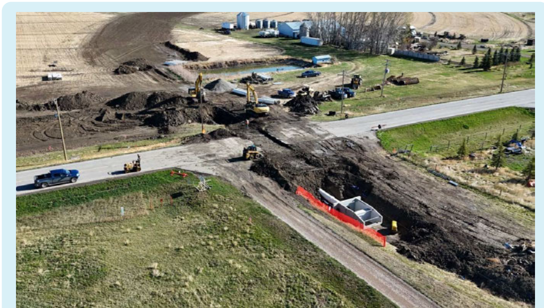
Lateral 61C Phase 1 – Kipp Road Crossing and Impact Baffle Structure Installation
