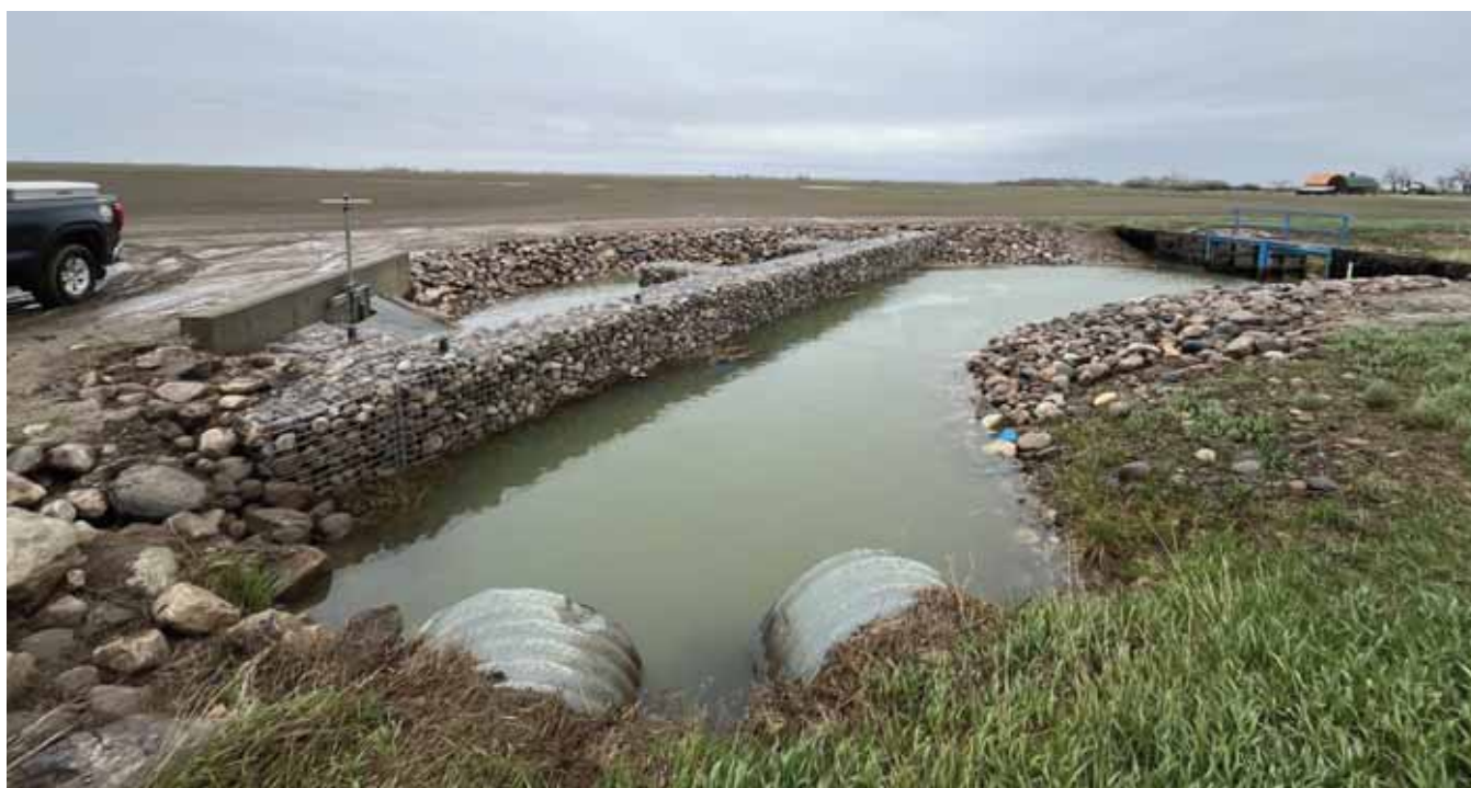
K4 Inlet Gabion - During Irrigation Season
