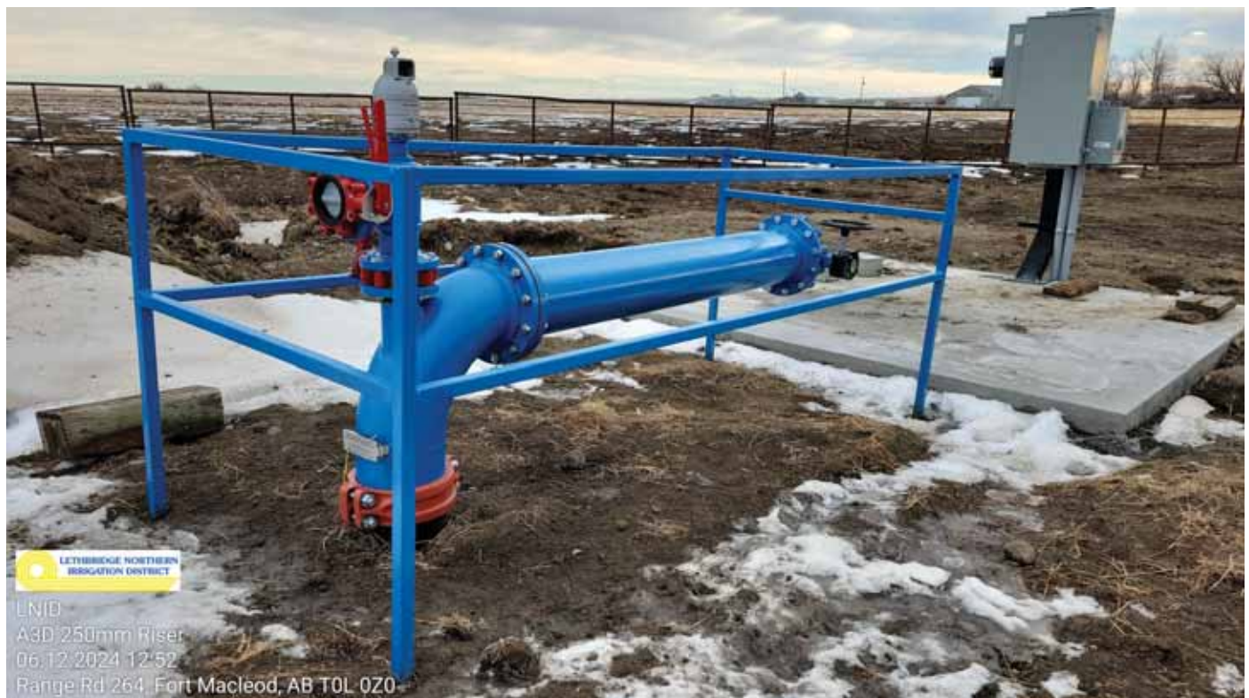
Lateral A3 – Newly Installed 10” Irrigation Turnout
