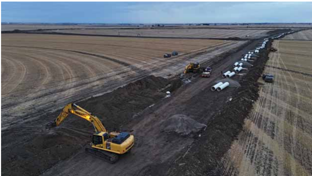
Lateral 61C – LNID Construction Crew Installing PVC Pipeline
