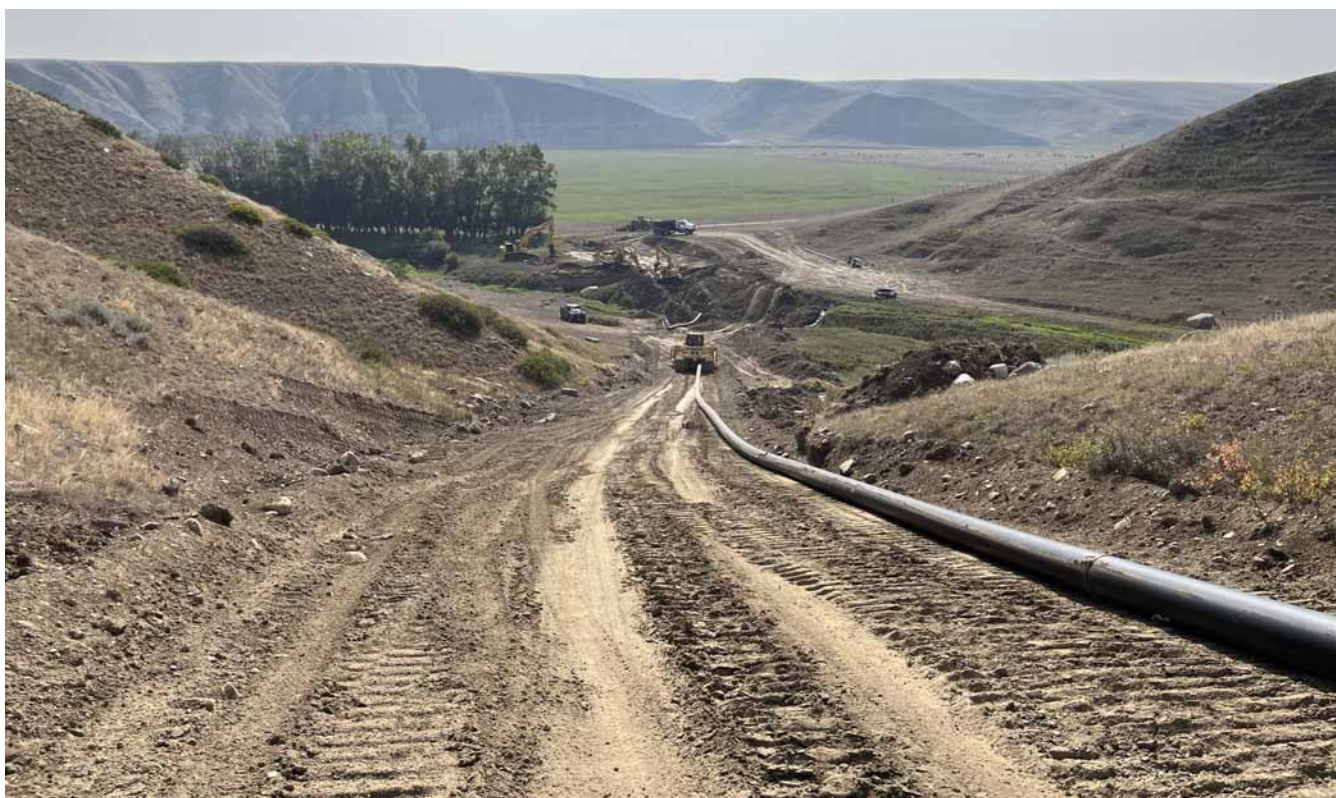
Lateral K2 - HDPE Pipe Installation
