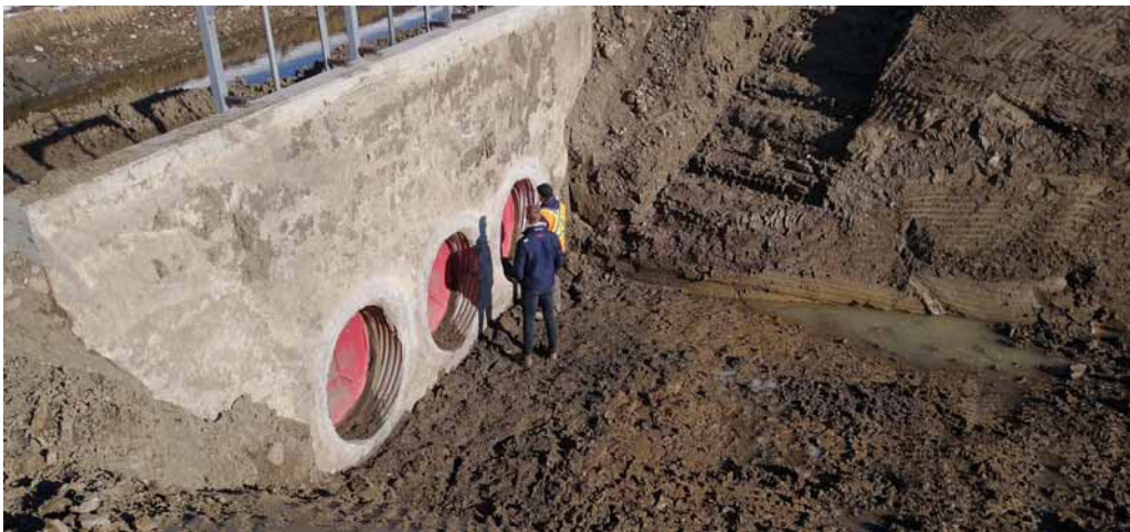
Lateral H3 Pond - 3 Inlet Pipes Removed
